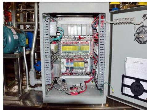
FWT Micro Pilot Unit control and data-logging system built by XRCC for hazardous location installation with over 60 instrument-loop input and outputs.
